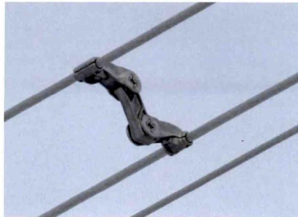
AltaLink is increasing inspections because installed spacer dampers of this type have failed on AltaLink transmission lines. Clamp bolts on the failed spacer damper did not remain secure and the clamp released from the wire, causing a portion of the spacer damper to fall to the ground. The picture below is an example of a spacer damper in a failed condition.
